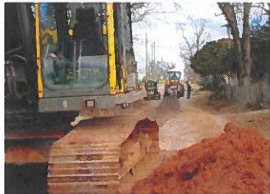
Figure 3. Construction along a residential street.
