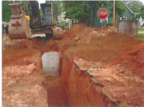
Figure 2. Installing a manhole for the new system
